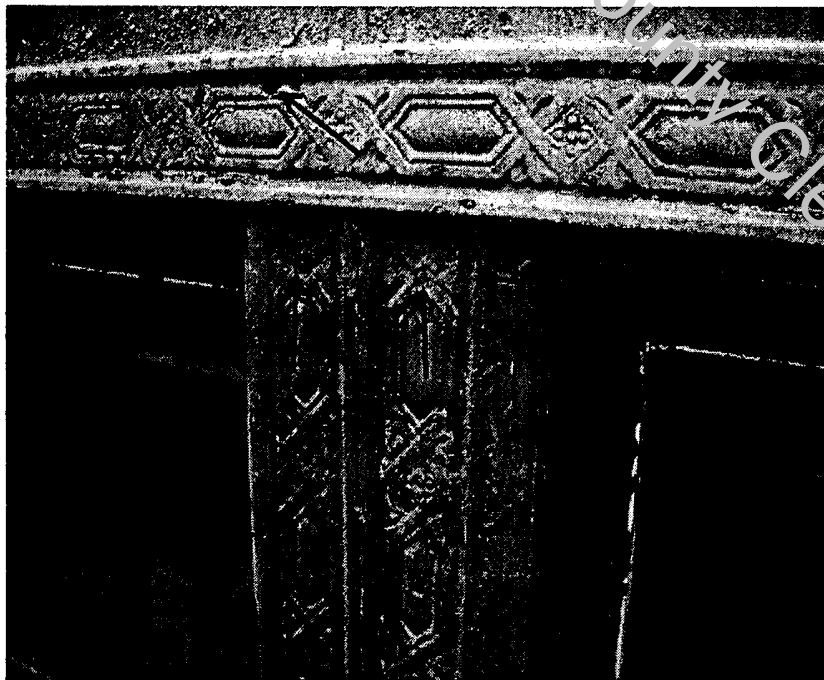
Figure 35 - Cast iron ornament at first floor installed during the 1986 renovation. Note deterioration of paint coating and corrosion beginning to bleed through coating. Arrows indicate fastener locations.
