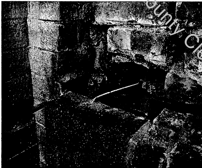
Figure 41 - New stainless steel lateral anchorage for decorative corner blocks above window. Rod was installed in epoxy filled hole on block and in epoxy in backup wall.
