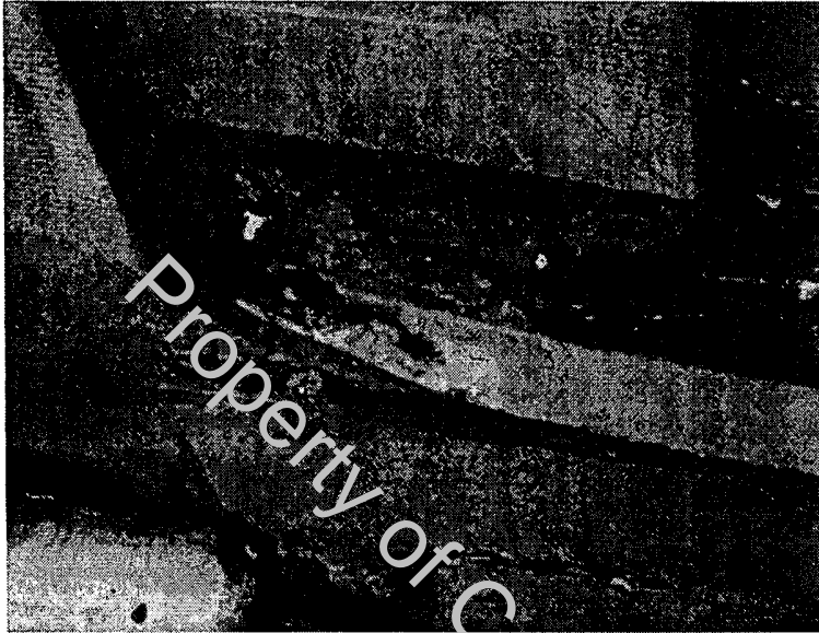
Figure 12 - Transition between 6th floor sheet metal and cast iron at 5th floor. Sheet metal sill laps over top edge of cast iron. Note corrosion of sheet metal sill at edges. This condition allows significant amount of water to enter the facade behind the cast iron.
